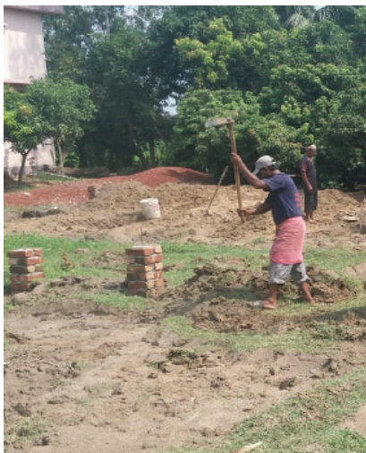
Temporary pillars to line up the building
